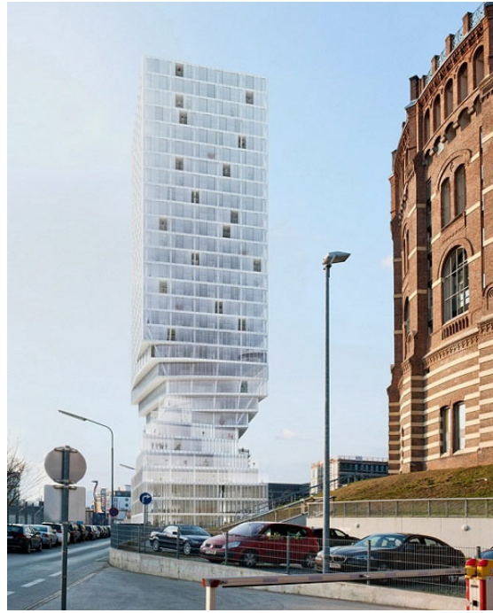
Figure 7. SEG Residential Tower in Vienna [9]
