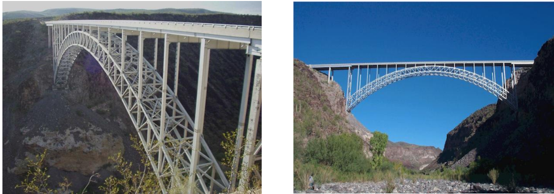
Figure 1. Burro Creek Bridge
